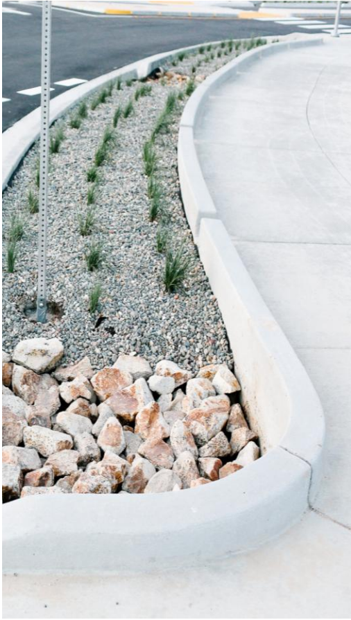
Bioswales Along the Roadside
