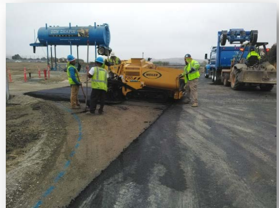
Crew prepares to expose manholes and water valves after mainline paving.
