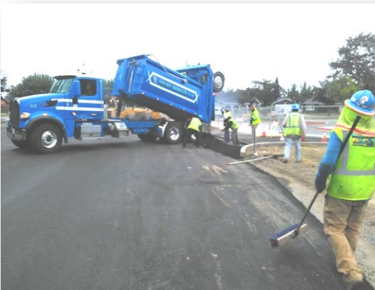
Crew prepares to expose manholes and water valves after mainline paving.
