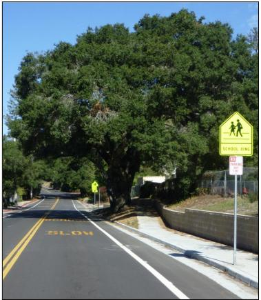
Mesiti-Miller Engineering prepared the design for the realignment and widening of 2,000 linear feet of Bean Creek Road between Scotts Valley Drive and Blue Bonnet Lane. The project added new bike lanes to each side of the road and new sidewalks to improve student safety and access to Scotts Valley Middle School.
