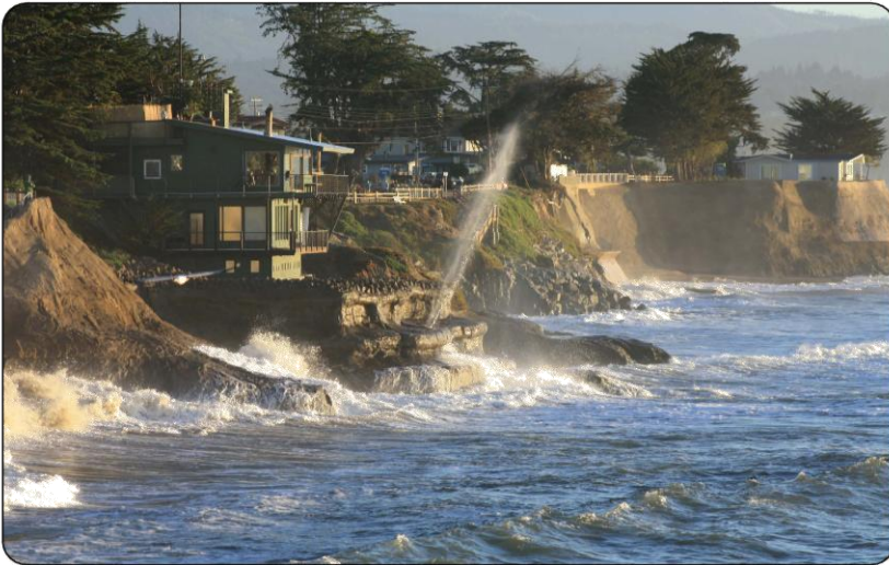
PRE-PLACED RIP RAP AGGREGATE
