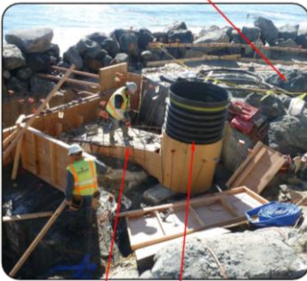
FLARED INLET VERTICAL CHAMBER WAVE ENERGY DISSIPATING CHAMBER UNDER CONSTRUCTION
