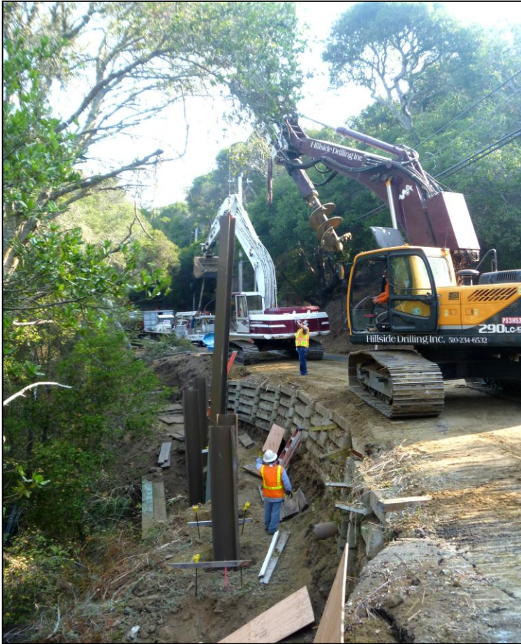
30ft-long steel piles were lowered into drilled holes to support the 18ft-tall, 100ft-long wall.
