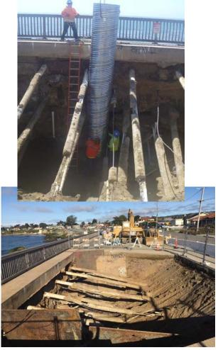
The 40 foot wide and 20 foot deep sinkhole opened up after a winter-long series of El Nino storms pushed heavy swells against the bluff, eroding the sandstone and protective boulders from below an existing retaining wall along West Cliff Drive.
