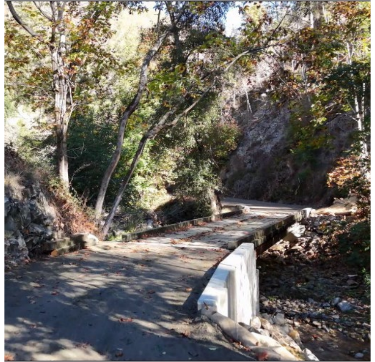
Completed Bridge Fall 2025
